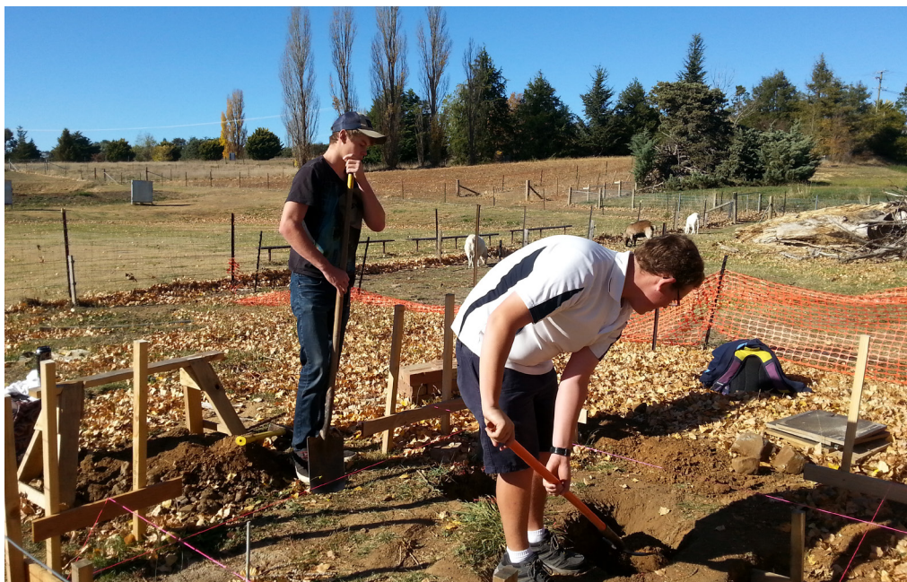
Construction students working on a project in the Monaro High School Agriculture plot.
